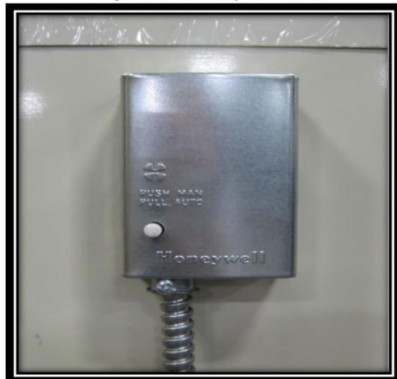
Fan/Limit Control, Mounted
