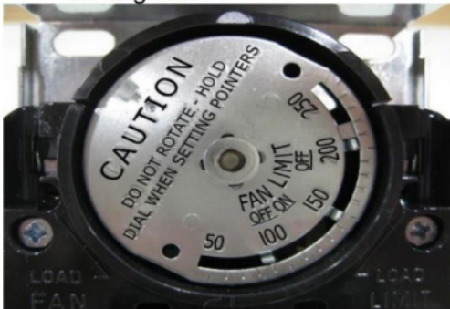
Fan/Limit Control Settings
